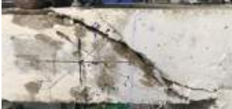
3.c) Final crack pattern of specimen (B3)
