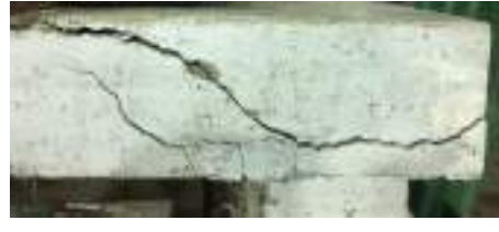
3.f) Final crack pattern of specimen (B6)
