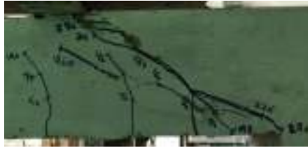
3.a) Final crack pattern of specimen (B1)
