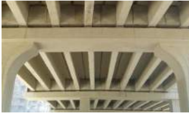
Figure 1: Wide shallow beams application in bridges
